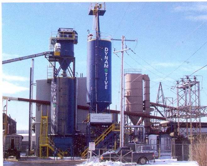
A Biomass plant
